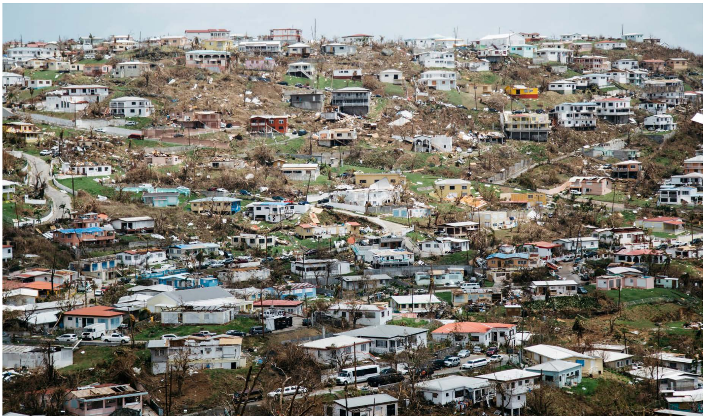
Damaged homes on St. Thomas Kareem Forbes
