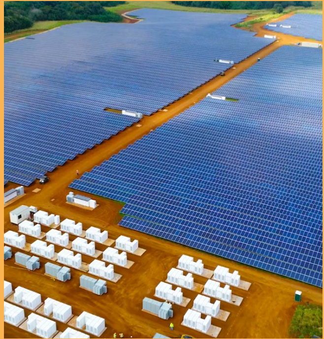
Solar panels coupled with battery storage in Kauai Tesla
