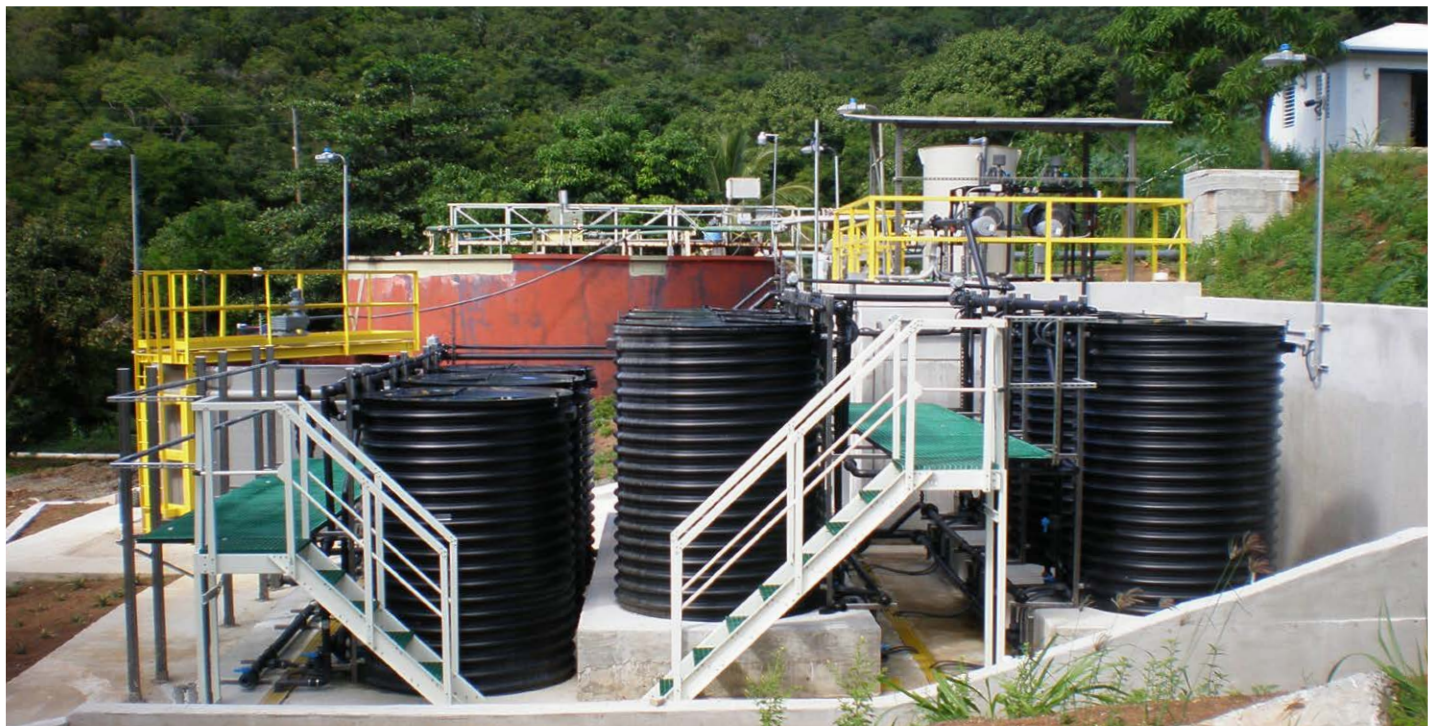
Bordeaux Wastewater Treatment Plant
