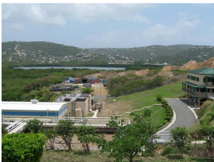
Mangrove Lagoon Wastewater Treatment Plant VIWMA
