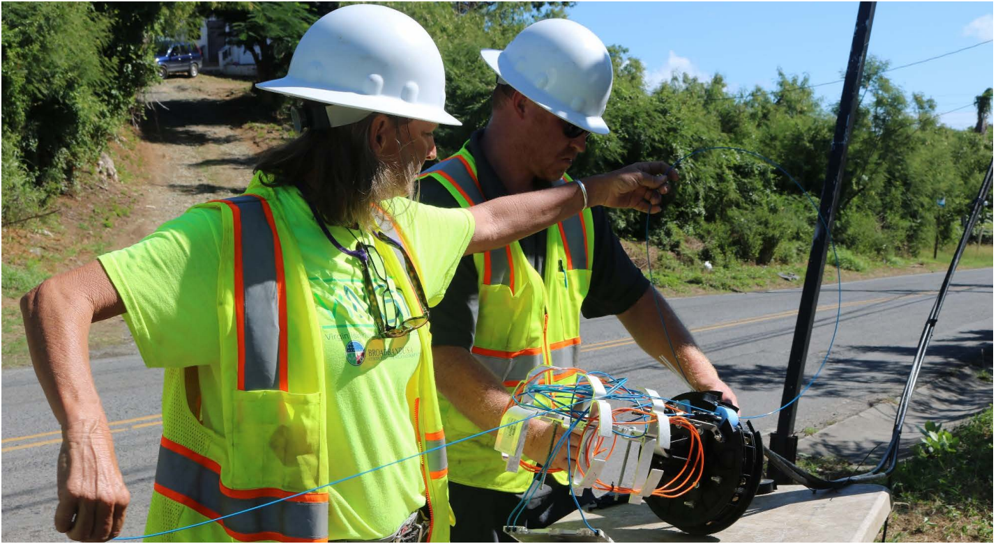
Crews repair damaged fiber lines viNGN
