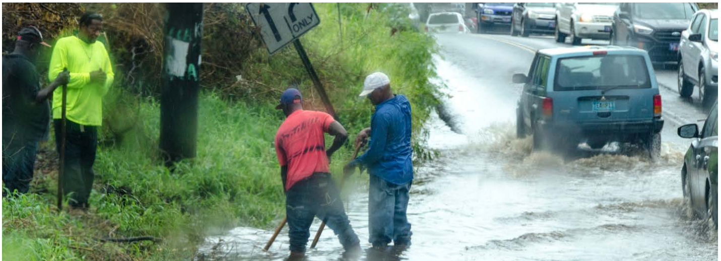
Workers clear debris from roadside drains during a rain storm to alleviate flooding on St. Thomas K.C. Wilsey/FEMA
