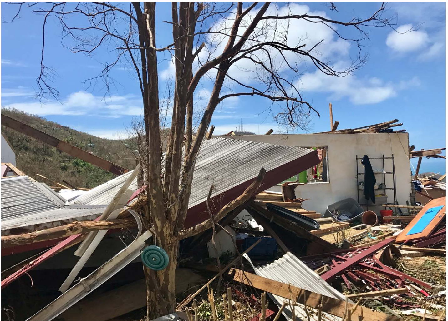
Destroyed home on St. Thomas after the hurricanes Kelsey Nowakowski
