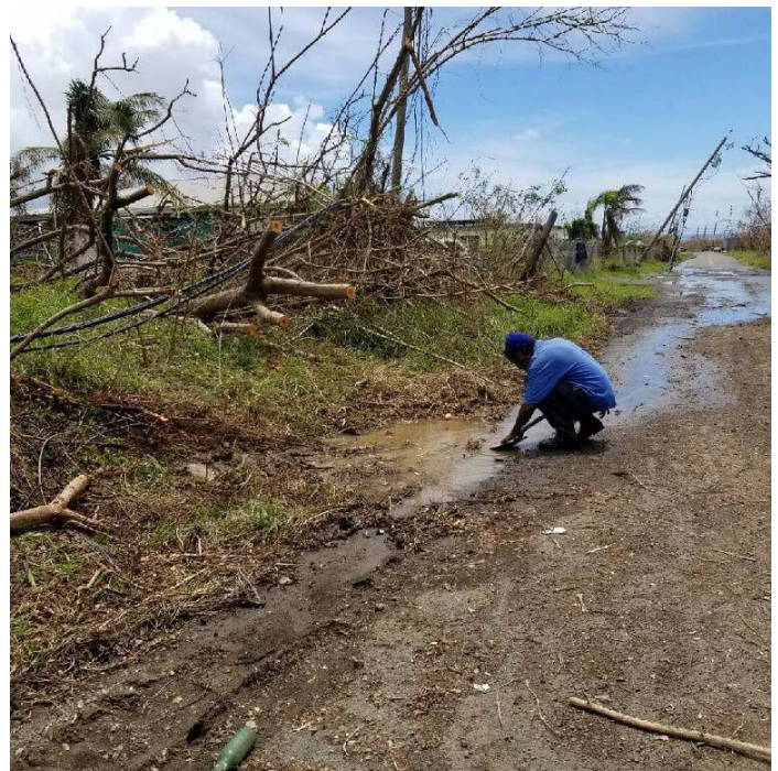
Water leak on St. Croix WAPA
